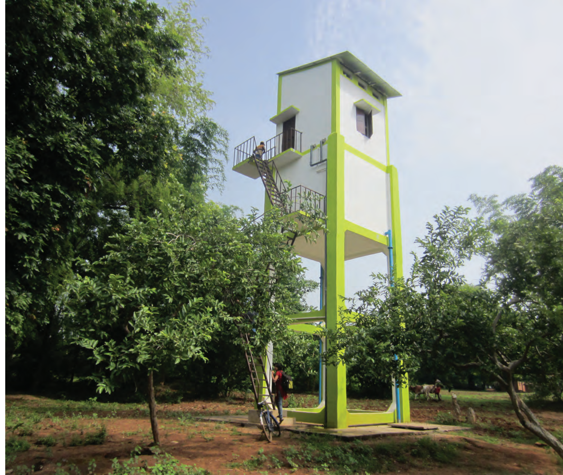
RIGHT: A newly completed AguaClara water tower stands in a rural village in Jharkand, India.
